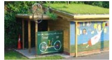
Green roof bike shelter by the Grass Roof Company.
